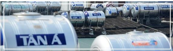
All of these tanks have a **Line in** to supply the tank with water and naturally a **Line out** to the building or house to supply water for daily use. As all the Lines-out are at the tank bottom, though the tanks are refilled daily. The water at the top of the tank is never used and becomes stagnant, the top water layer can become a breeding ground for
